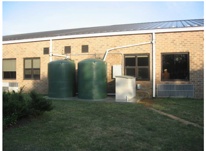
A larger rain harvesting system at Samuel Mickle School in East Greenwich, NJ. The collected water is pumped through an irrigation system that supplies an ornamental garden. Photo credit: Elaine Rossi-Griffin, Rutgers Cooperative Extension.
