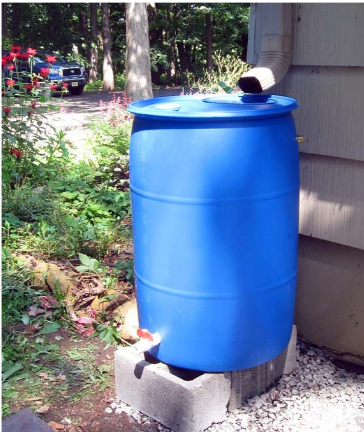
A rain barrel collects water from the roof of a house. The water is then used to irrigate ornamental plantings. Photo credit: Michele Bakacs, Rutgers Cooperative Extension.
